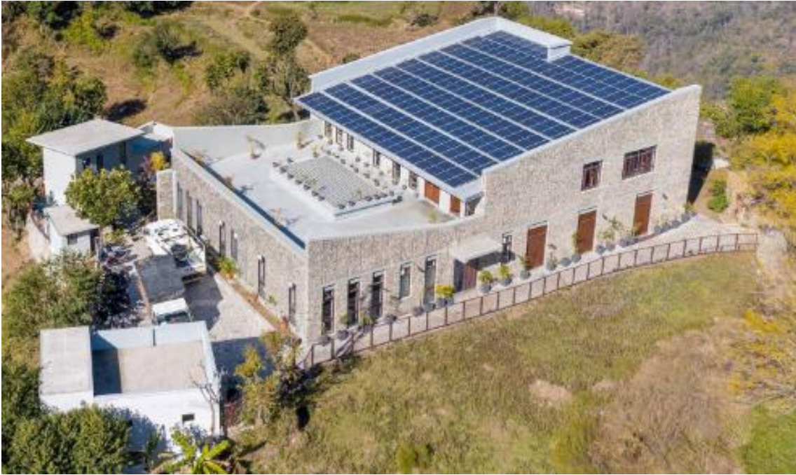
A 50 kWp Solar Roof installed on the building (source: Abdel, 2019).
