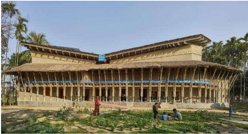
Anandaloy building (source: nzeb.in).
