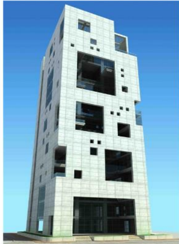
Mobil House, Dhaka, Bangladesh (source: nzeb.in)
